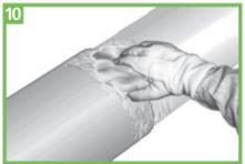
Final cleaning of the sealing surface to remove the loose HDPE and sand particles caused by the roughening with a dry, grease- and lint-free cloth.
