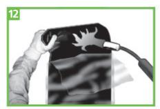
Cut off the corners of the sleeve approx. 20 x 50 mm on one side for later underlapping. Pull the separatig film approx. 15 cm from the end of the shrink sleeve (underlap) and briefly heat the hot-melt adhesive with the propane flame.
