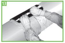
Place the end of the Superseal product centrally over the socket pipe/joint casing transition area and perpendicular to the pipe axis approximately on the apex of the pipe, press the heated area firmly with the heel of your hand.
