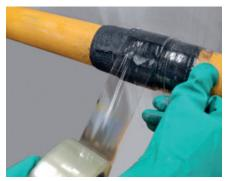
**6.** Overwrap with clear foil or adhesive tape tightly
