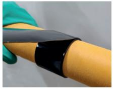
**3.** Remove sanding residue and wrap anti-sliding tape with 100% overlap in required layers
