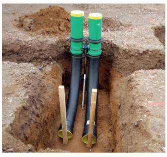
The new district heating baseplate penetration 4 pipes has been developed for direct concrete encasing into the baseplate, for the feed-in and secure sealing of flexible district heating pipes. The components can be mounted in just a few simple steps:
