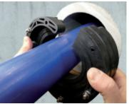
5. Push the seal on the carrier pipe.
