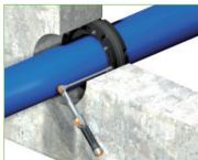
7. Use a torque wrench to tighten the nuts according to the below table.
