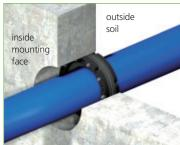
6. Insert the Pressio® seal into the wall and place it flush with the outside of the building.
