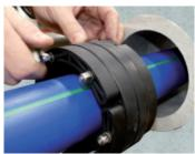
6. Reassamble the Pressio® seal on the carrier pipe.
