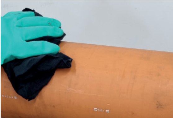
1. Clean pipe surface, dry, degrease
