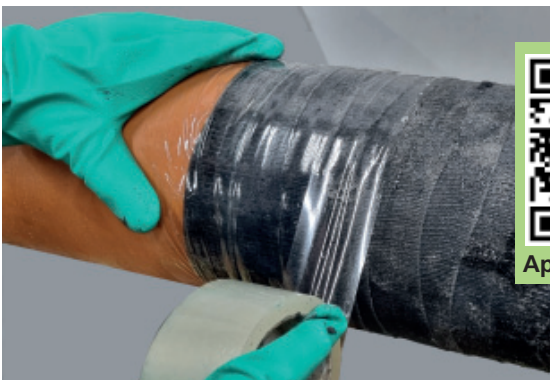
5. Overwrap with clear foil or adhesive tape tightly
