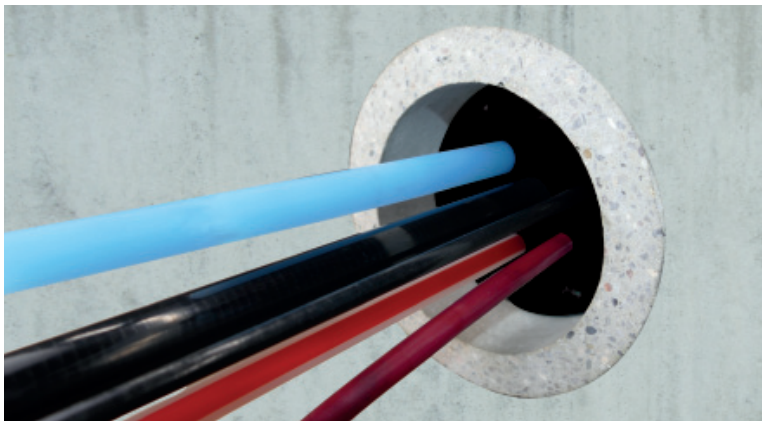
Standard 4 cables® FIXED closed/split without blind plugs
