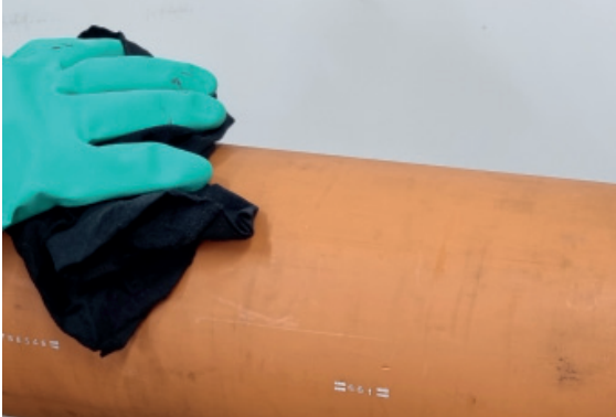
1. Clean pipe surface, dry, degrease
