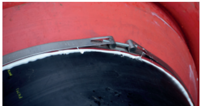
4 pipes stainless steel straps used for pipe sizes up OD 315 mm Torque value 10 Nm
