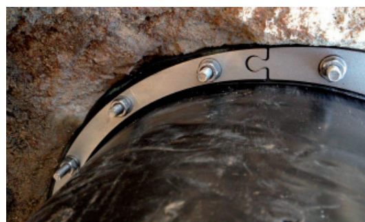
Pressio® individual, split, potable water, non centric
