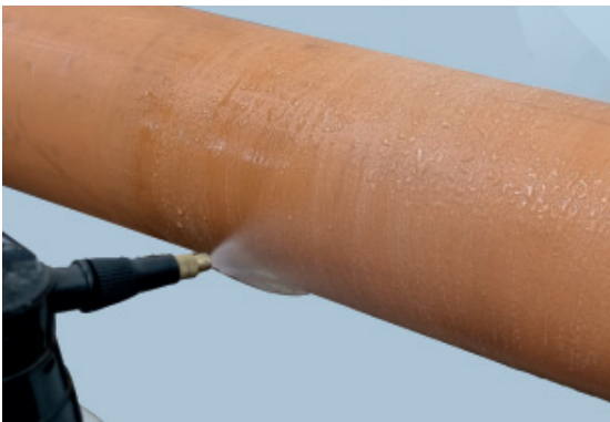
3. Remove sanding residue and moisten surface
