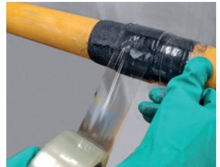
6. Overwrap with clear foil or adhesive tape tightly
