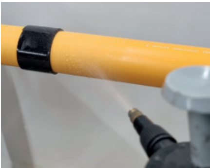
4. Moisten surface incl. anti-sliding tape
