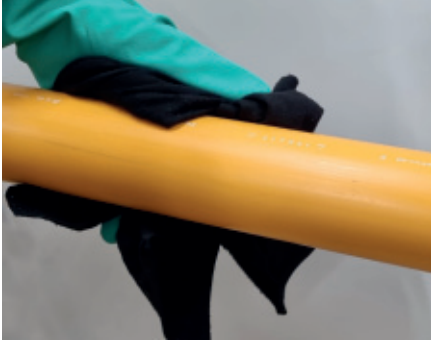
1. Clean pipe surface, dry, degrease
