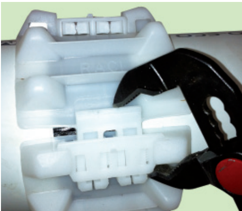
Assembly with F/G tightening lever
