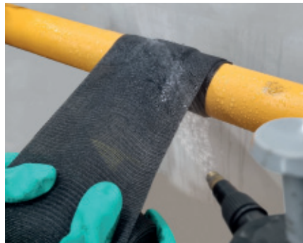
5. Wrap the Pipecoat Plus tape with 100% overlap in required layers. Spray water on the tape continuously during the wrapping process. Time of processing 2-3 min., depending on temperature
