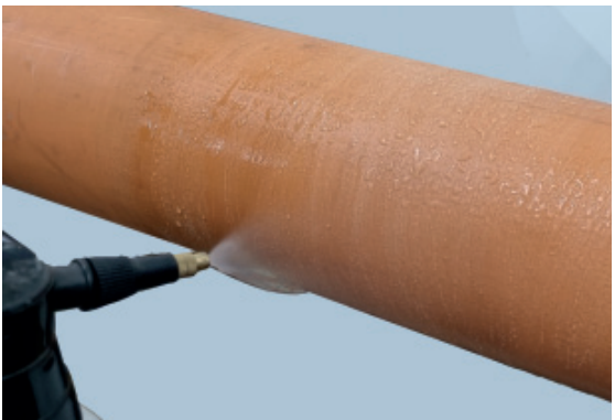
3. Remove sanding residue and moisten surface
