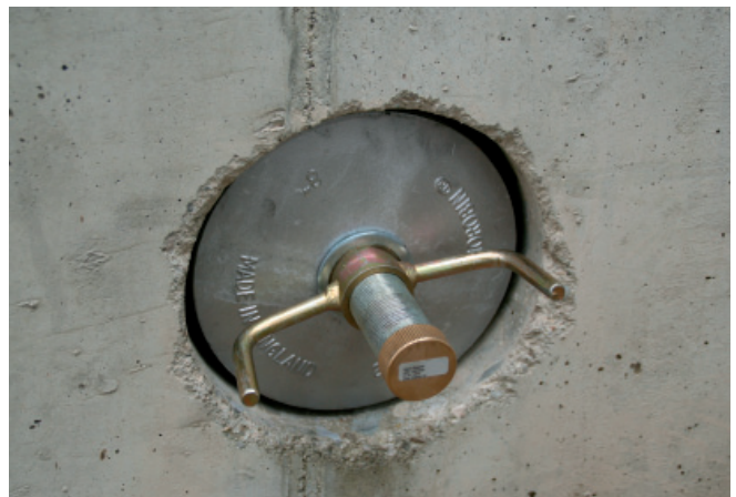
Aqua Stopper closes core drilled hole
