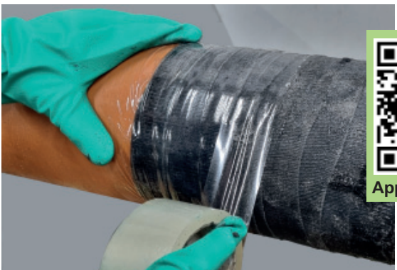
5. Overwrap with clear foil or adhesive tape tightly
