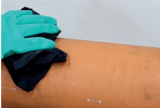
1. Clean pipe surface, dry, degrease
