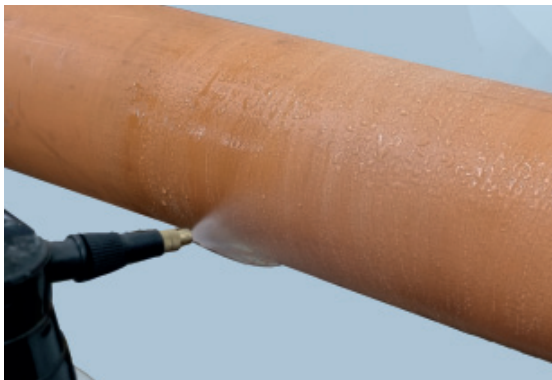
3. Remove sanding residue and moisten surface
