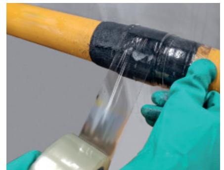
6. Overwrap with clear foil or adhesive tape tightly
