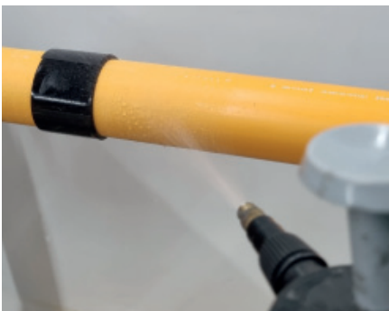
4. Moisten surface incl. anti-sliding tape
