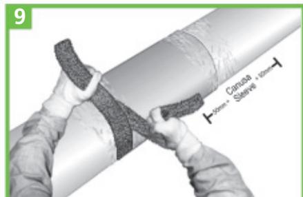
Roughen the sealing surface with emery cloth (grain 40-60), approx. 50 mm wider than the shrink sleeve.
