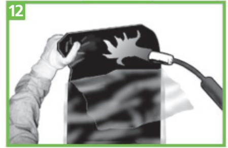
Cut off the corners of the sleeve approx. 20 x 50 mm on one side for later underlapping. Pull the separating film approx. 15 cm from the end of the shrink sleeve (underlap) and briefly heat the hot-melt adhesive with the propane flame.
