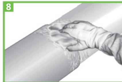
Degreasing the sealing surface with PE cleaner resp. ethanol/spirit (min. 94%) and a dry, grease- and lint-free, non-staining cloth.
