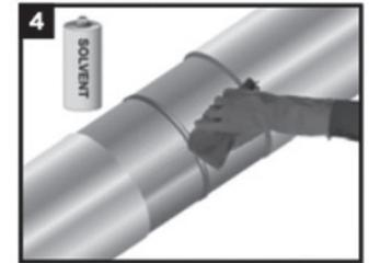
Ensure that the PE coating edges are beveled to 30°. Clean exposed steel and adjacent pipe coating with a solvent cleanser to remove the presence of oil, grease, and other contaminants.
