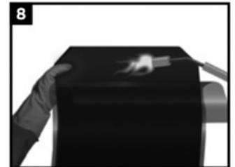
As an option, slightly trim corners of pre-attached closure. Partially remove the release liner and gently heat the underlap approximately 150 mm (6") from the edge.
