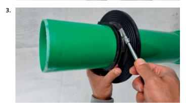
Fasten steel straps on both sides around the wall collar.
