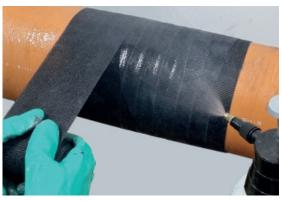
**4.** Wrap the Pipecoat Plus tape with minimum 1 x 75 % overlap (4 layers). **Spray water on the tape continuously during the wrapping process**. Time of processing 2-3 min., depending on temperature
