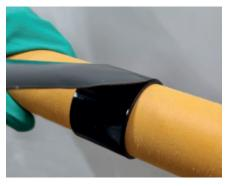
**3.** Remove sanding residue and wrap anti-sliding tape with 100% overlap in required layers
