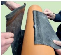
After the adhesive on the bonding strips has dried sufficiently, the AKO end seal is wrapped around the carrier pipe.
