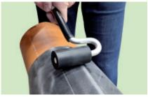
Align the two bonding strips over each other and press them firmly together.
