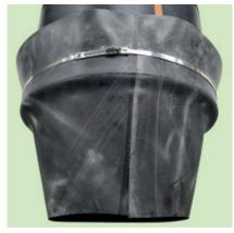
The larger end of the casing end seal is pulled onto the casing pipe until it is tightly in position. A stainless steel tensioning strap is then used to hold the end seal in place on the casing pipe.
