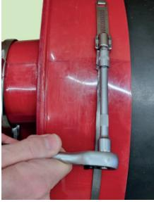
4. Fasten the casing end seal on the carrier pipes and the casing pipe with the tightening straps.
