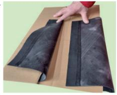
The AKO casing end seal has to be prepared on a clean surface, with its two tapered bonding strips facing upwards.
