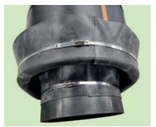
After that, the end seal should be tucked in and then fastened securely to the carrier pipe using another stainless steel tensioning strap.
