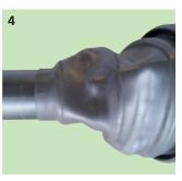
4. After that, push AWM-seal over carrier pipe and casing pipe.
