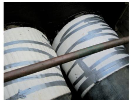
Before backfilling protect sealing sleeves with expansion-pads
