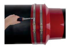
4. Fix second strap with 10 Nm (smoothen escaping sealant). Repeat step 2 to step 4 on the carrier pipe
