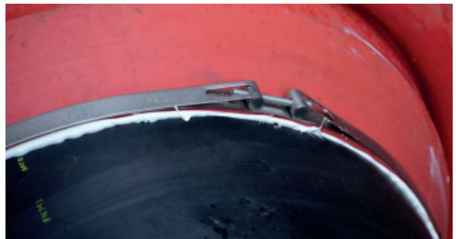
4 pipes stainless steel straps used for pipe sizes up **OD 315 mm**
