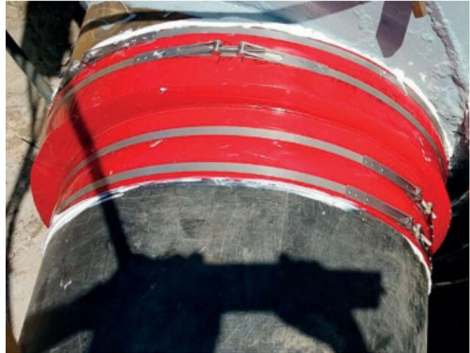
**Pipe movements and subsidence** are the big challenges for a **pipeline wall penetration seal**, especially at **pre-insulated high-temperature pipelines**.
