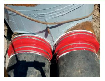
**Pipe movements and subsidence** are the big challanges for a **pipeline wall penetration seal**, especially at **pre-insulated high-temperature pipelines**.
