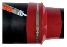
3. Fill the sealant all around under the sleeve
