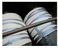
Before backfilling protect sealing sleeves with expansion-pads
