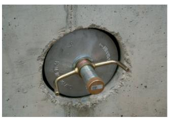
Agua Stopper closes core drilled hole
